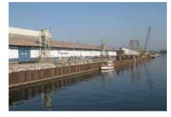
PZ 35 steel sheet pile section 16 meters (52.5 feet) long provided by Skyline Steel at A572-60 steel grade.
